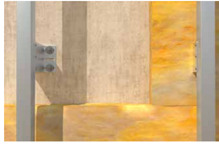
Façade substructure
