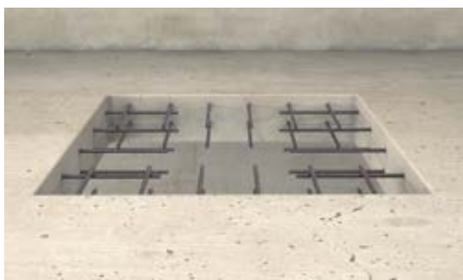
Closing a ceiling opening
